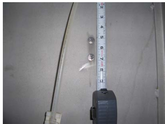
Holes for water manifold mounting U-Bolts, 5-1/4" and 7-3/4" from top of cabinet
