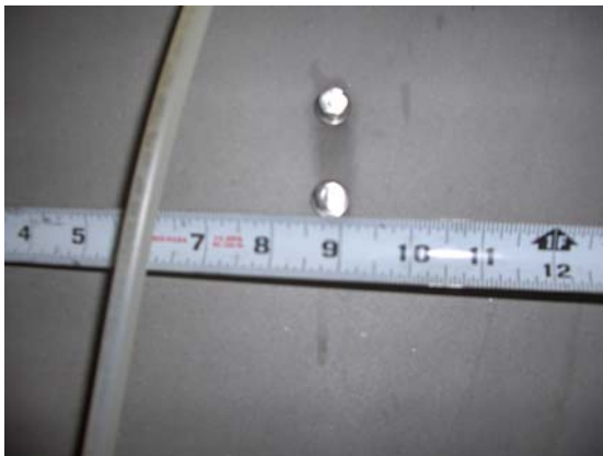
1-3/4" water inlet hole centered between frame angles, 11-1/2" from each angle
