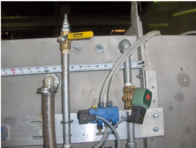
1-3/4" water inlet hole centered between frame angles, 11-1/2" from each angle
